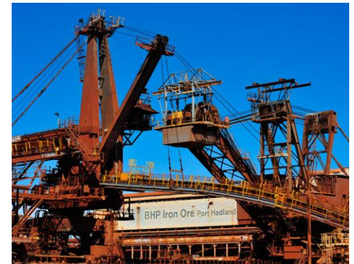
BHP Iron Ore Port Hedland
