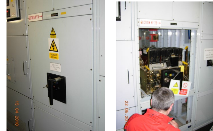
Before: obsolete Square D circuit breakers
