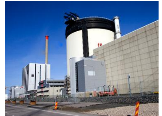
Ringhals TR3 Reactor
